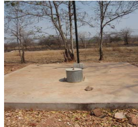
Burial pits constructed for waste disposal at Mola District Hospital.
